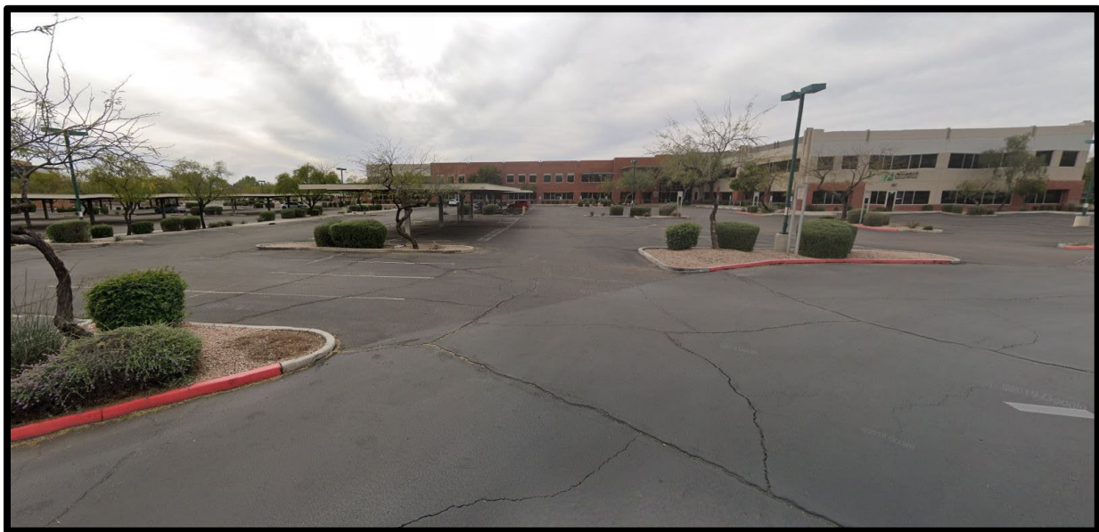
Figure 2 Existing Property looking west (Source: Google Street view dated March 2019)
